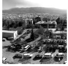
UNITED STATES VEMBASSY NEW BUILDINGS Athens, Greece Project Phase > Preliminary and Final Design Review - Specifications - Building Permit Revision Total Area > 13,500 m 2 Owner > Embassy of the United States of America Client > United States department of State
