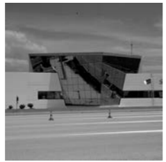
RIO-ANTIRIO BRIDGE OPERATIONS MANAGEMENT BUILDING Western Greece Project Phase > All Phases Total Area > 2,102 m 2 Client > GEFYRA S.A.
