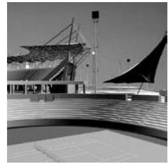
ATHENS OLYMPIC TENNIS CENTRE Marousi, Athens, Greece Project Phase > Detailed Design - Architectural Competition Total Area > 23,000 m 2 Owner > General Secretariat of Athletics Client > GEK S.A.
