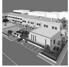
TECHNICAL PROFESSIONAL SCHOOL Kalambaka, Greece Project Phase > Preliminary Design - Competition Total Area > 3,500 m 2 Client > Prefecture of Trikala - Technical Department
