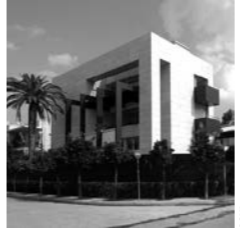
FILOTHEI RESIDENCE CONTEMPORARY LUXURY RESIDENCE Filothei, Athens, Greece Project Phase > All Phases Total Area > 384,00 m 2 Owner > NAT S.A.
