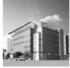
I.K.A. SERVICES BUILDING Thessaloniki, Greece Project Phase > Preliminary Design - Competition 2nd Place Total Area > 8,500 m 2 Client > IKA Department of Construction and Housing
