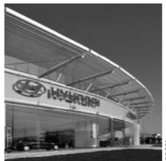
OFFICES & AUTO SHOW MIXED USE RETAIL COMPLEX Attica, Greece Project Phase > All Phases Total Area > 7,890 m 2 Owner > THISEUS S.A. Client > Private Client
