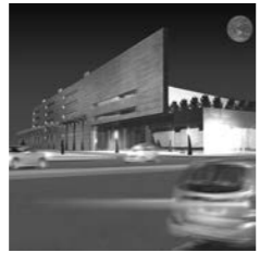
PIRAEUS BANK OFFICE AND RETAIL BUILDING COMPLEX Athens, Greece Project Phase > Competition - Preliminary Design Total Area > 39,300 m 2 Client > PIRAEUS BOTIFIN S.A.
